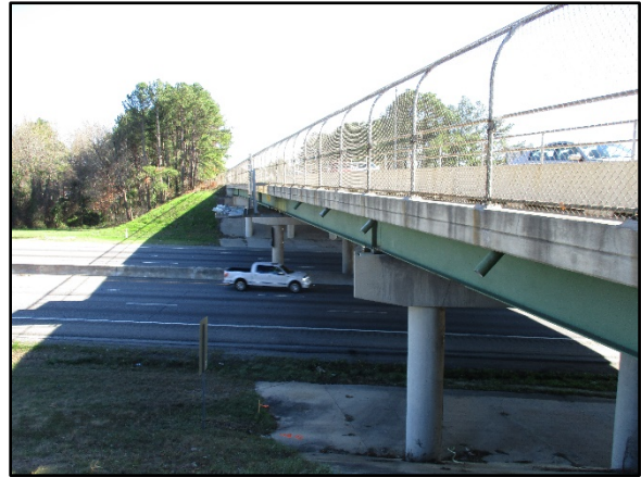
Photo 1 – S-40-757 (Harbison Blvd) Bridge over I-26 in Richland County, SC.
